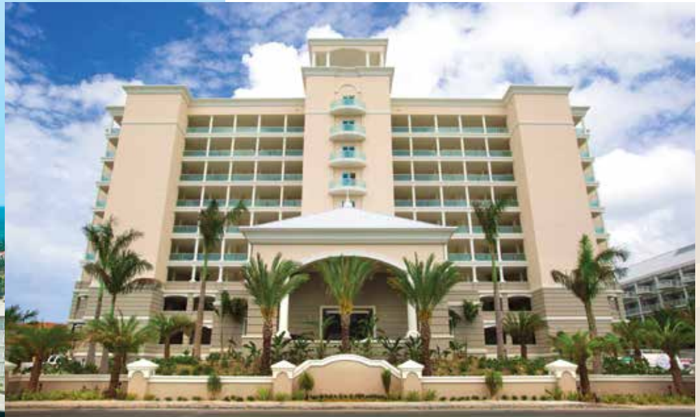
The WaterColours residences on Seven Mile Beach is among a growing number of high-end developments taking shape in Cayman.
